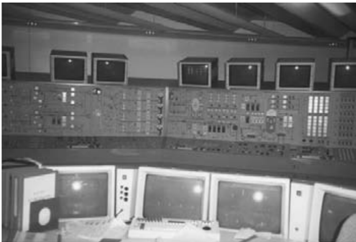
Figure 13.2 The experimenter's view of a nuclear power plant control room simulator (reproduced by permission of British Energy)
